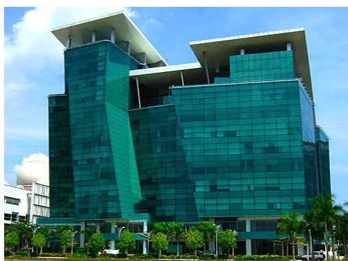
Figure 2c – Modern commercial buildings (Putrajaya): High window-to-wall ratio (note most blinds are drawn down)
